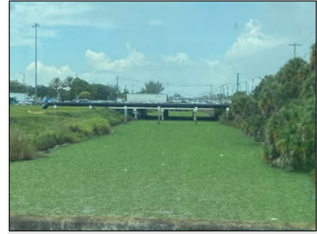
Figure 7-37. Water lettuce clogging a canal in Palm Beach County (photo by SFWMD).
