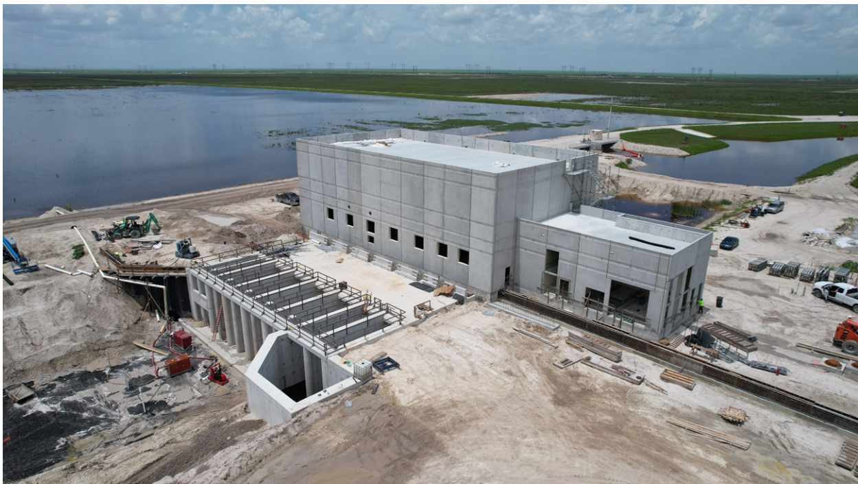
Figure 5A-3. STA-1W Expansion #2. View of G-781 construction (photo by SFWMD in 2023.)
