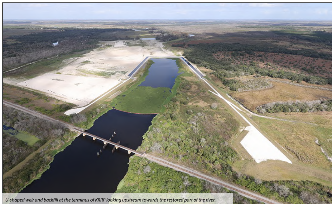
U-shaped weir and backfill at the terminus of KRRP looking upstream towards the restored part of the river.
