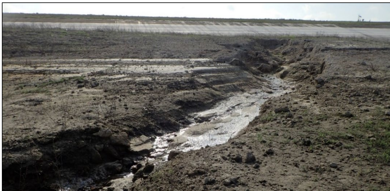
Figure 18. Southern bank of Cell 6 in the L-8 FEB on April 14, 2020
