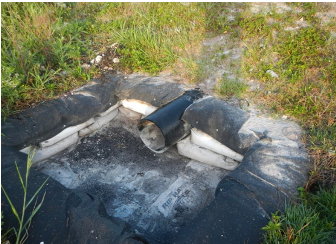
Figure 3. An outflow sump installed in all test cells. (Photo by SFWMD.)
