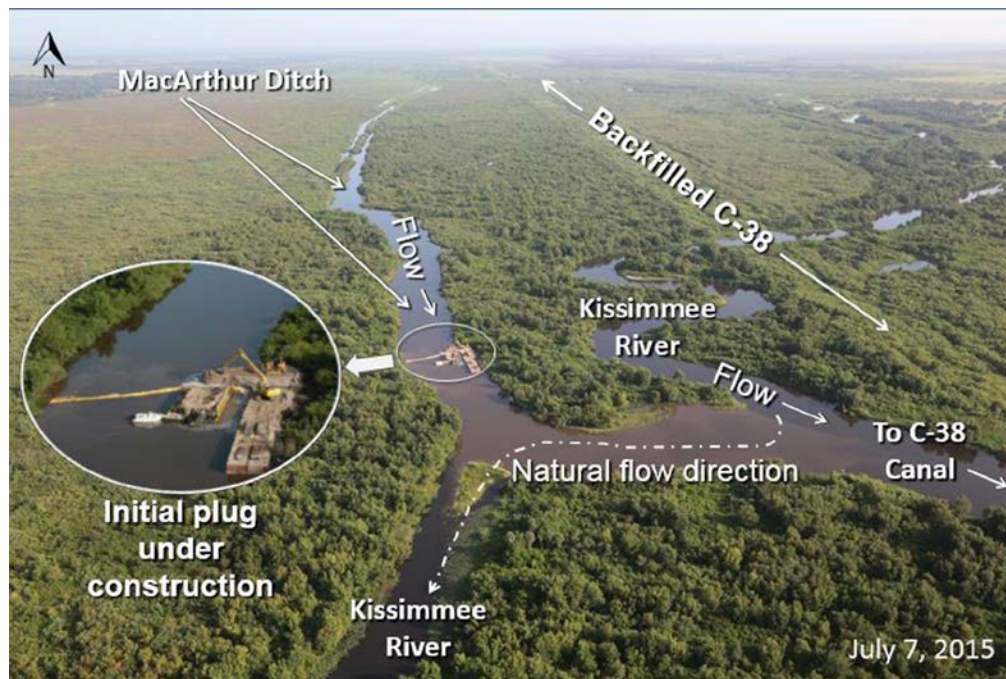
Figure 9-34. KRREP Phase I restoration area MacArthur Ditch Backfill Project.
