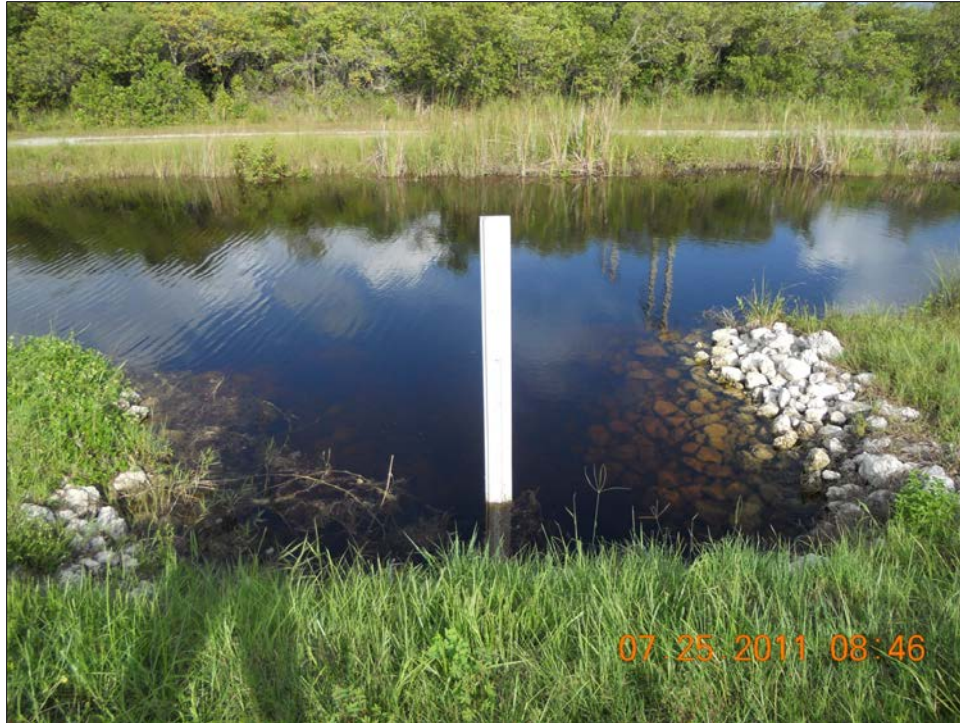
Figure C-5. Staff gauge upstream of culvert S-23A.
