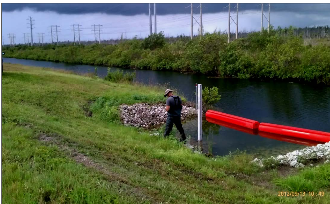
Figure C-2. Upstream L-31E culverts after repairs.
