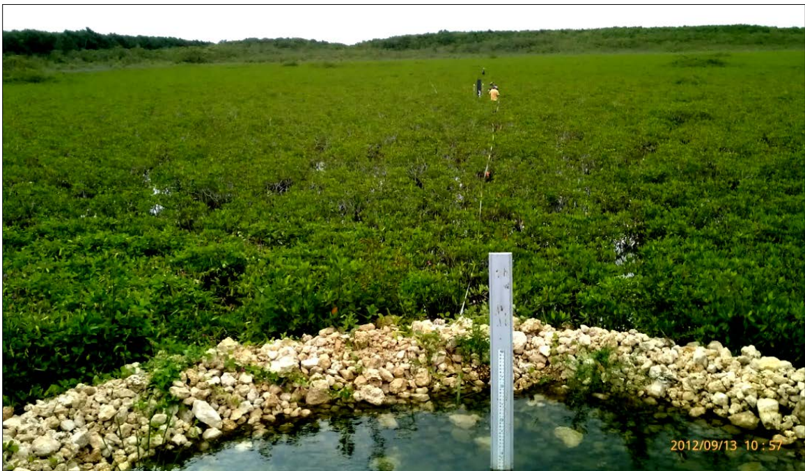
Figure C-4. Downstream L-31E culverts after repairs.
