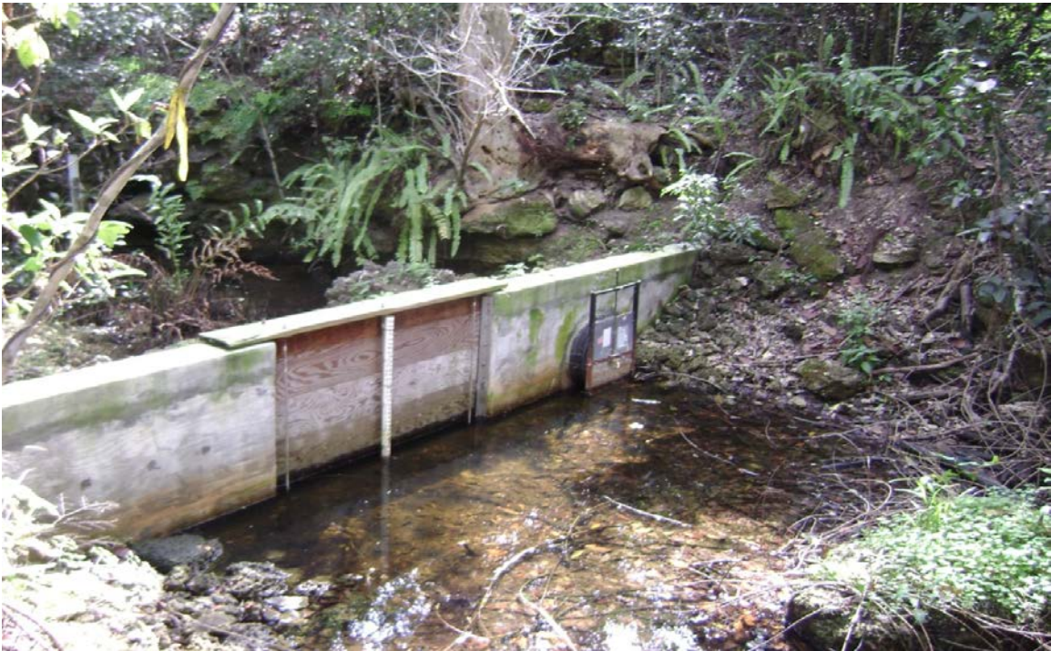
Figure A-6. Close-up of the upstream side of the weir in Cutler Creek.
