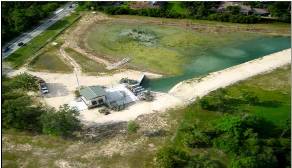
Figure A-2. Pump station S-700 and educational wetlands.
