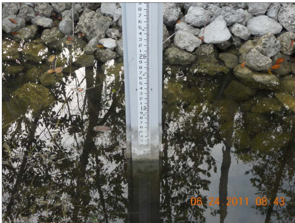
Figure C-6. Staff gauge downstream of culvert S-23A.
