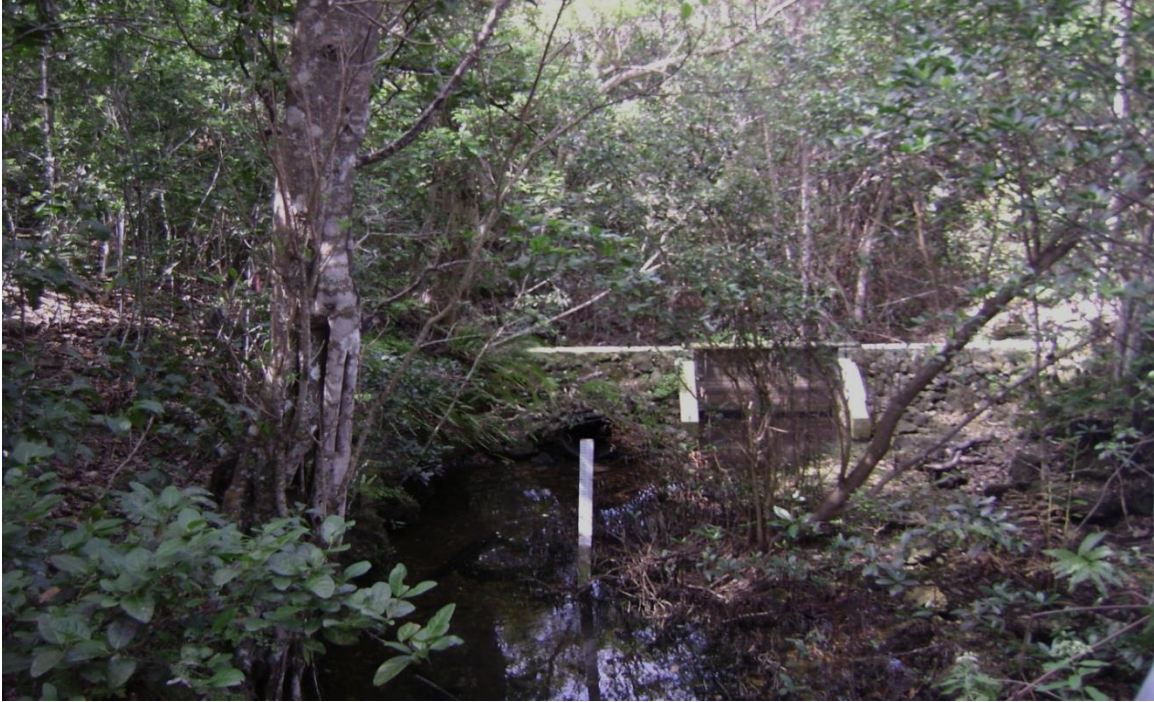
Figure A-5. Existing wetland staff gauge 3 within Cutler Creek upstream of the weir.
