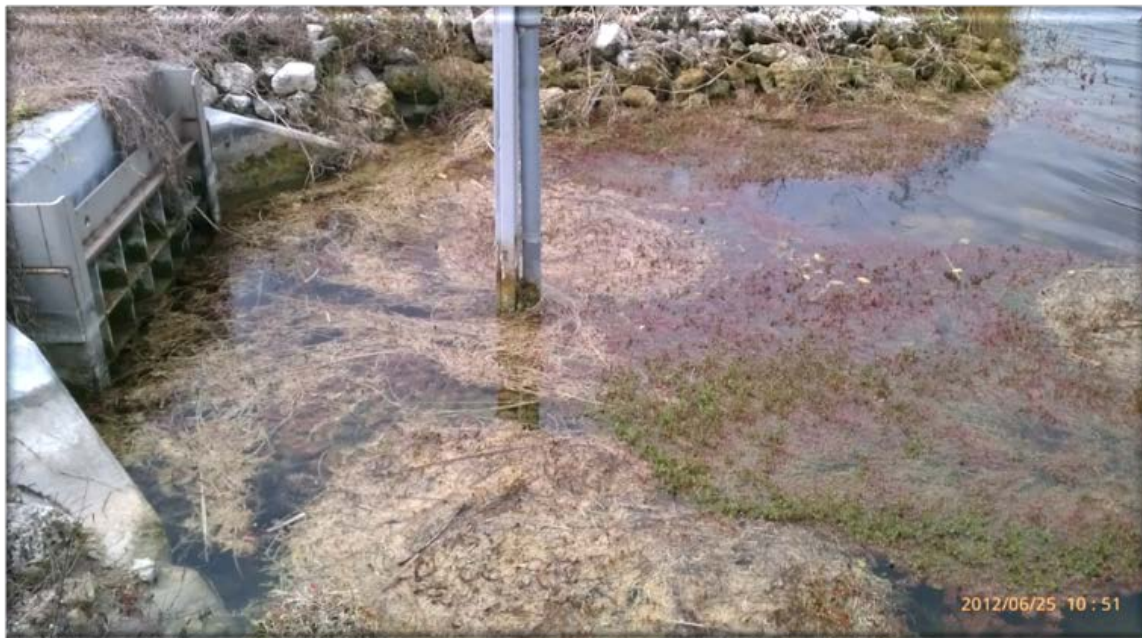
Figure C-1. Upstream L-31E culverts before repairs.
