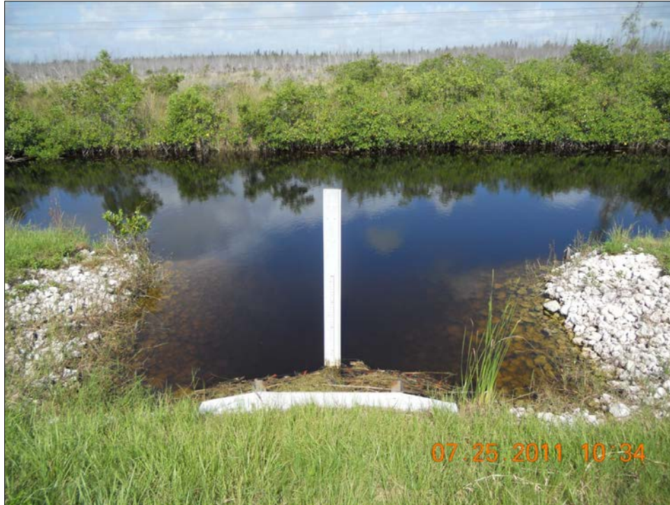
Figure C-9. Staff gauge upstream of culvert S-23D.
