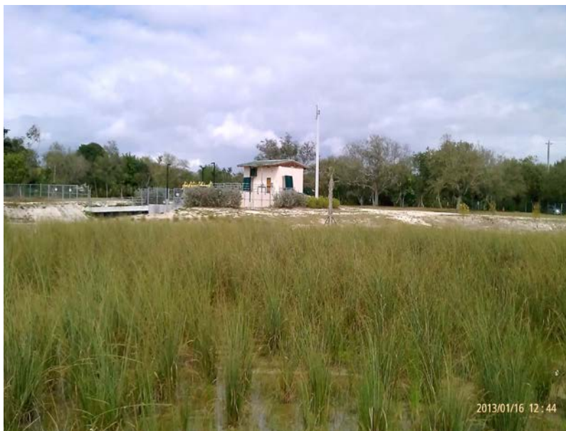
Figure 1. Pump station S-700 constructed for the BBCW Deering Estate Flow-way.
