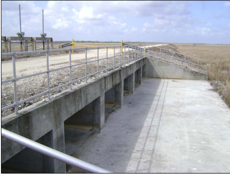
Figure 37. Westerly view of the G-423 Interbasin Transfer Structure discharge.
