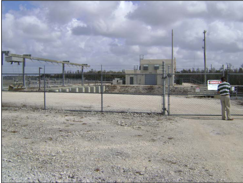
Figure 25 . Northerly view of the G-422 Intake Pump Station.
