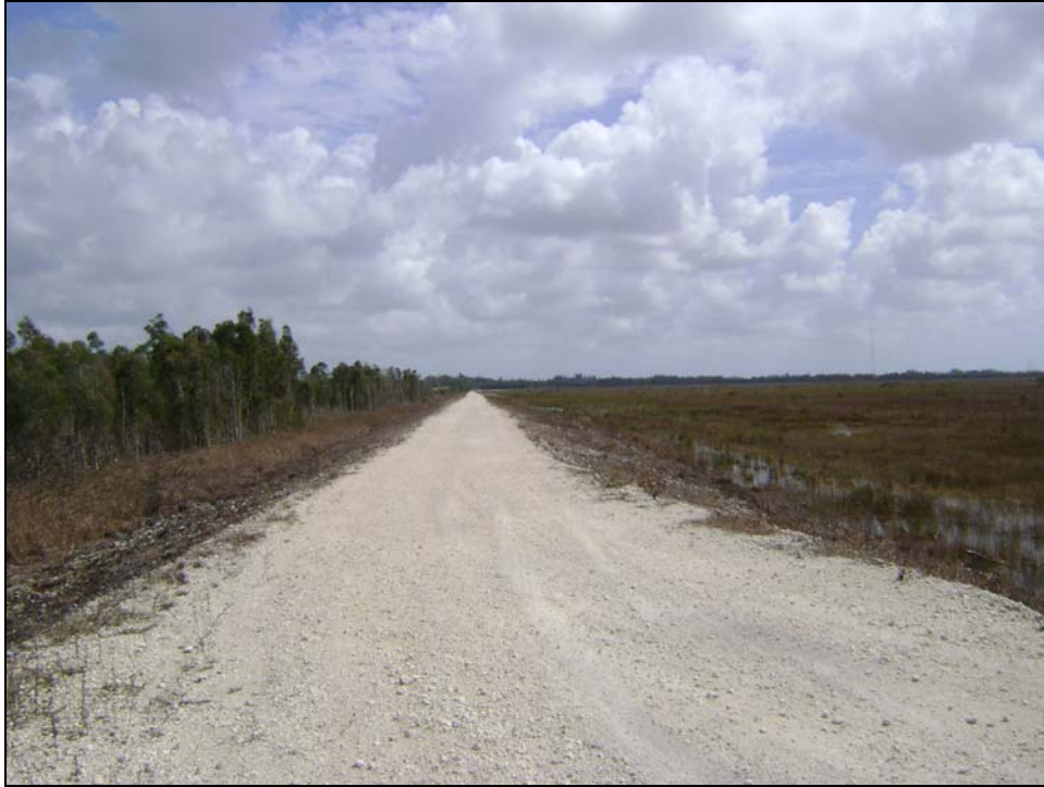
Figure 13. Easterly view of the North Cell North Perimeter Levee as seen from the northwest corner of the Basin. At this corner the levee top transitions into a 25 to 30-foot wide West Perimeter levee. The inside and outside slopes are 4H:1V and 2.5H:1V, respectively. Sparse withered vegetation noted. No ruts or erosion was observed.
