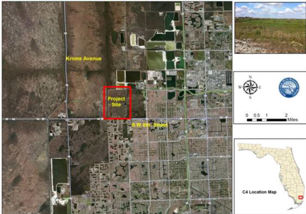
Figure 1. Overview of the C-4 Emergency Detention Basin (C-4 EDB).
