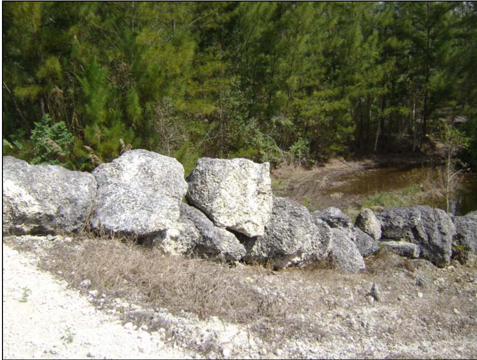
Figure 9. Northeasterly view of the 3-foot boulders installed at the northeast corner of the North Cell to prevent motorized vehicles from entering the C-4 Emergency Detention Basin.
