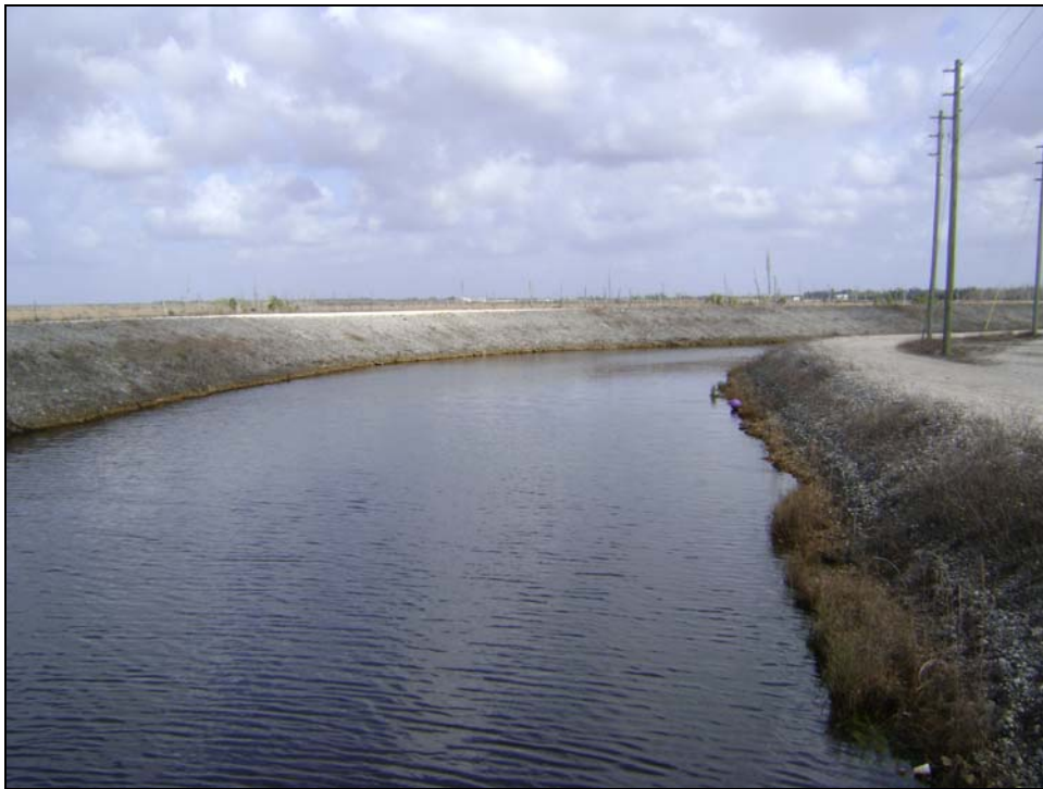
Figure 38. Northerly view of the Supply Canal as seen from the access bridge. There are no erosion or slope failure observed on the canal banks.
