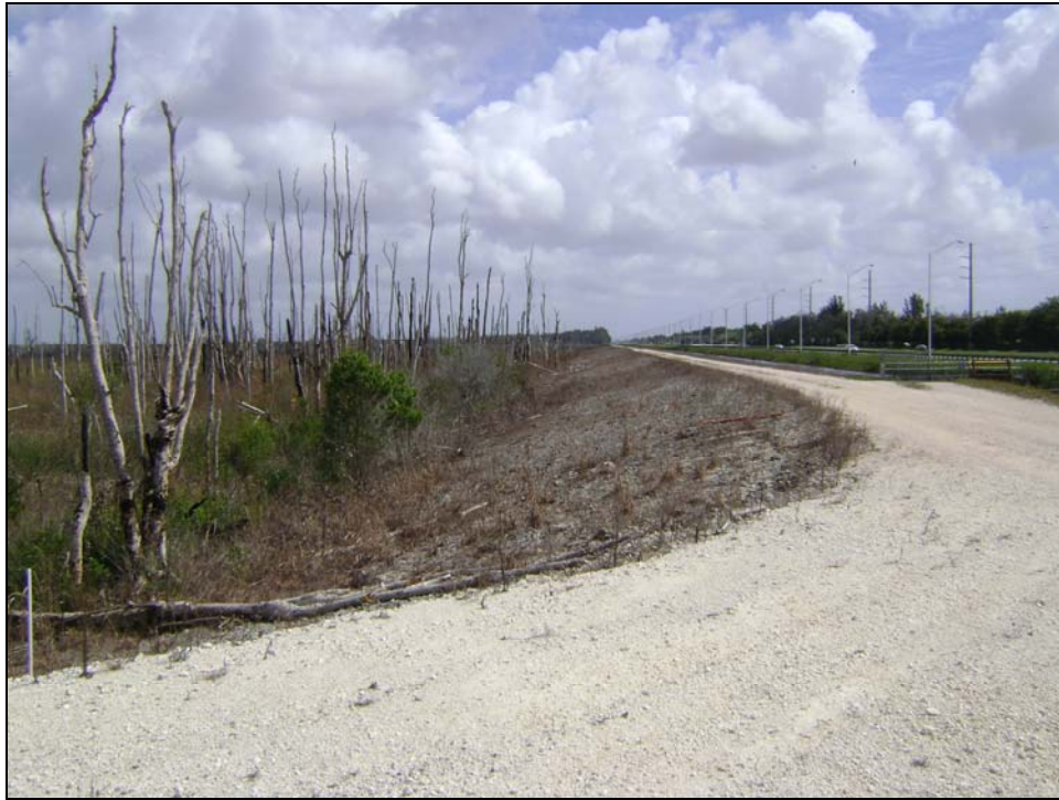
Figure 21. Easterly view of the 14-foot wide South Cell South Perimeter Levee as seen from southwest corner. The inside and outside slopes are 4H:1V and 2H:1V, respectively. Sparse withered vegetation noted. No ruts or erosion was observed.
