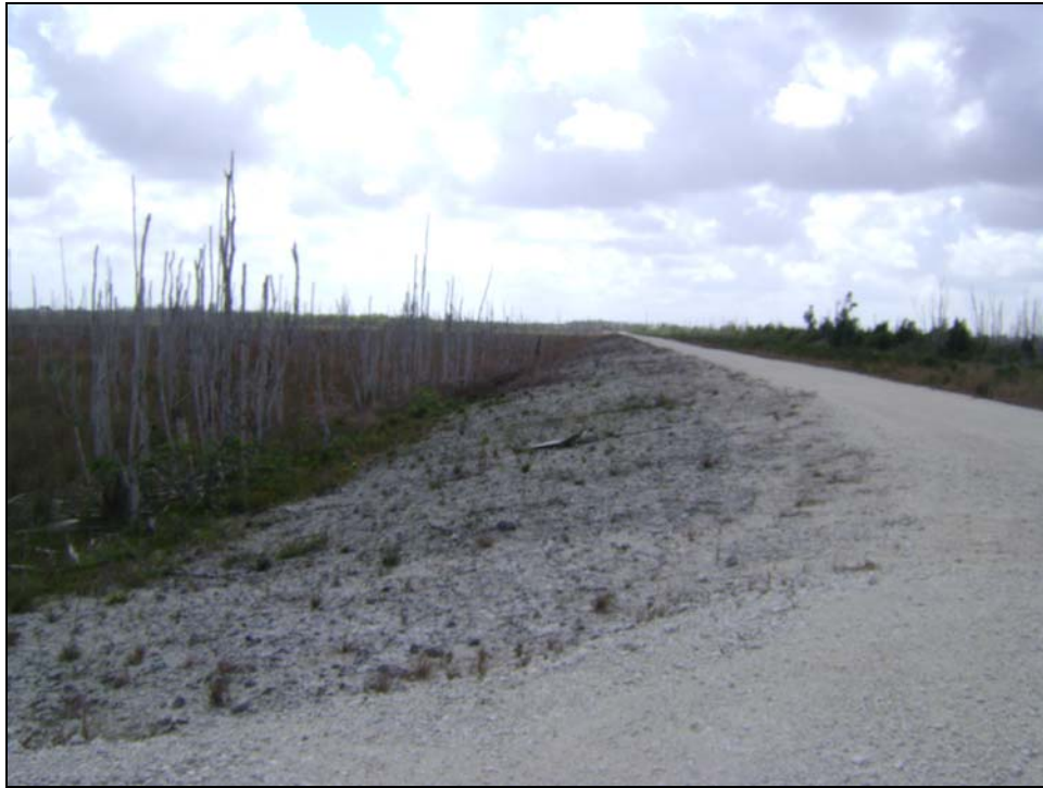
Figure 19. Southerly view of the 14-foot wide South Cell West Perimeter Levee as seen from its junction with the Interior Levee. The inside and outside slopes are 4H:1V and 2H:1V, respectively. Sparse withered vegetation noted. No ruts or erosion was observed.
