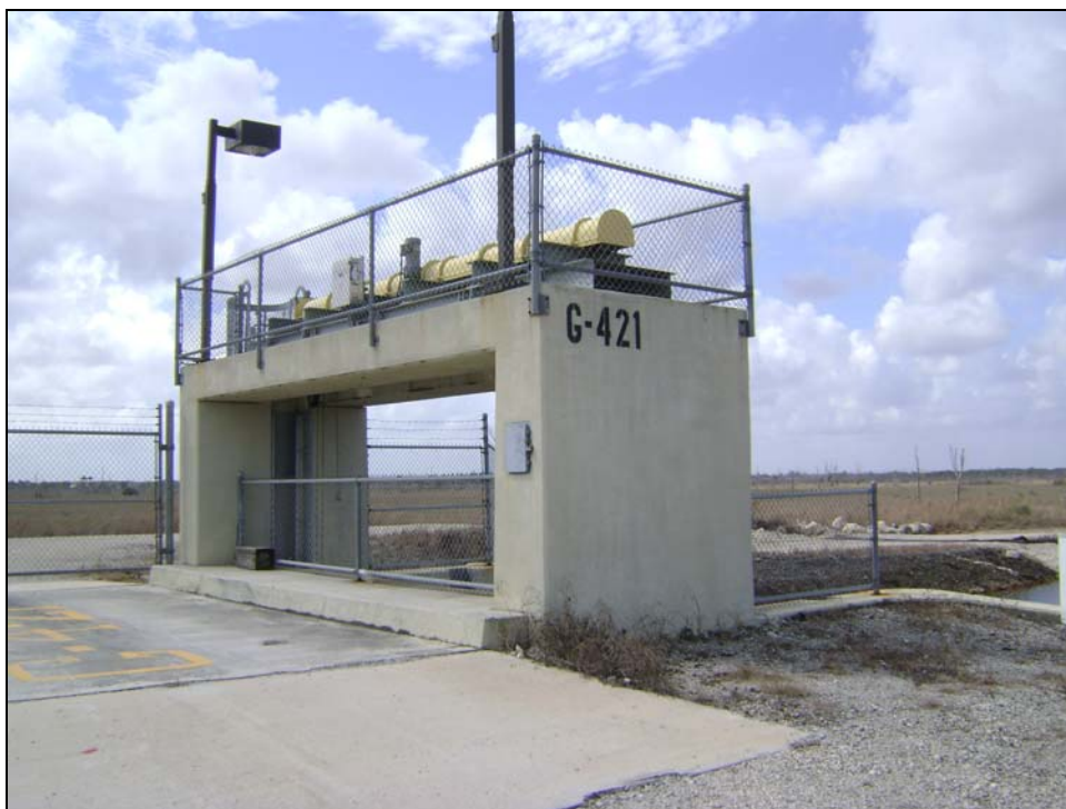
Figure 30. View of the G-421 Gated Spillway Structure service bridge. No cracks observed on the concrete surfaces.
