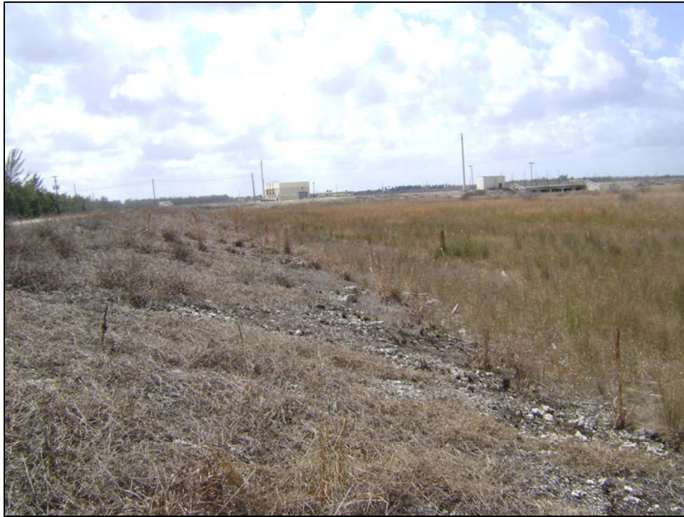
Figure 7. Southerly view of the North Cell Perimeter Levee inside slope 0.2 miles north of the intersection of the Interior Levee and the North Perimeter Levee. The 4H:1V inside slope has a mixture of 6" muck and limestone gravel and boulders with withered vegetation cover. No ruts or erosion was observed.
