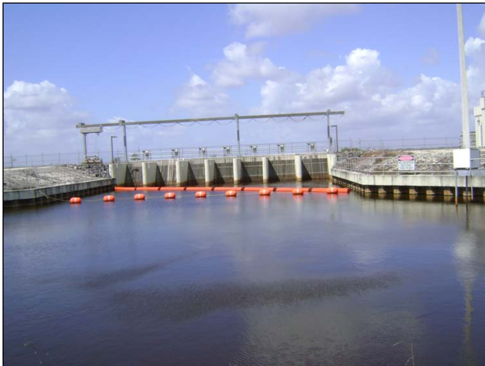
Figure 26. Westerly view of the G-422 Intake Pump Station showing the trash rake system and seven pump bays with 89cfs electric pumps. The concrete abutments and steel sheet pile walls are in good condition.
