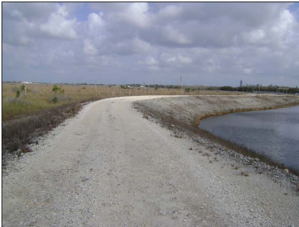
Figure 4. Northerly view of the 14-foot wide East Perimeter Levee and the Supply Canal from the southeast corner of the South Cell. The inside and outside slopes are 4H:1V and 2.5H:1V, respectively. The majority of the side slopes are bare of vegetation. The weeds on the slopes are withered. No ruts or erosion was observed.
