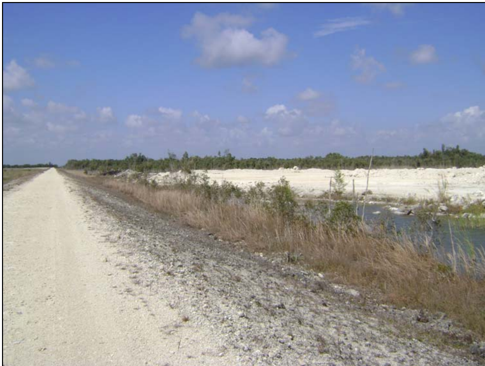
Figure 12. Westerly view of the North Cell North Perimeter Levee and the CEMEX Mines, 0.4 miles west of the northeast corner of the Basin. The inside and outside slopes are 4H:1V and 2.5H:1V, respectively. Sparse withered vegetation noted. No ruts or erosion was observed.
