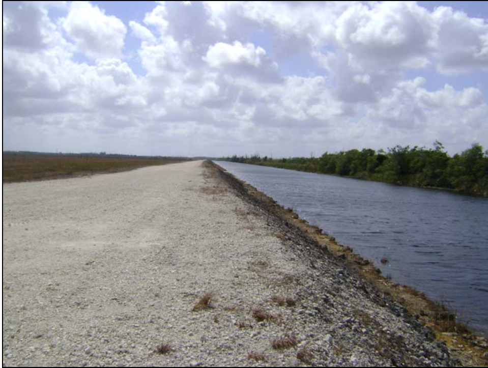
Figure 15. Southerly view of the North Cell West Perimeter Levee and Borrow Pit as seen from the northwest corner. The outside slope is 1H:1V. Sparse withered vegetation noted. No ruts or erosion was observed.
