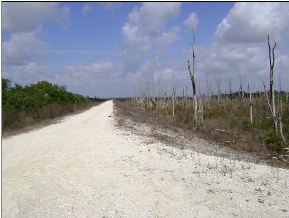
Figure 20. Northerly view of the 14-foot wide South Cell West Perimeter Levee as seen from the southwest corner. The inside and outside slopes are 4H:1V and 2H:1V, respectively. Sparse withered vegetation noted. No ruts or erosion was observed.
