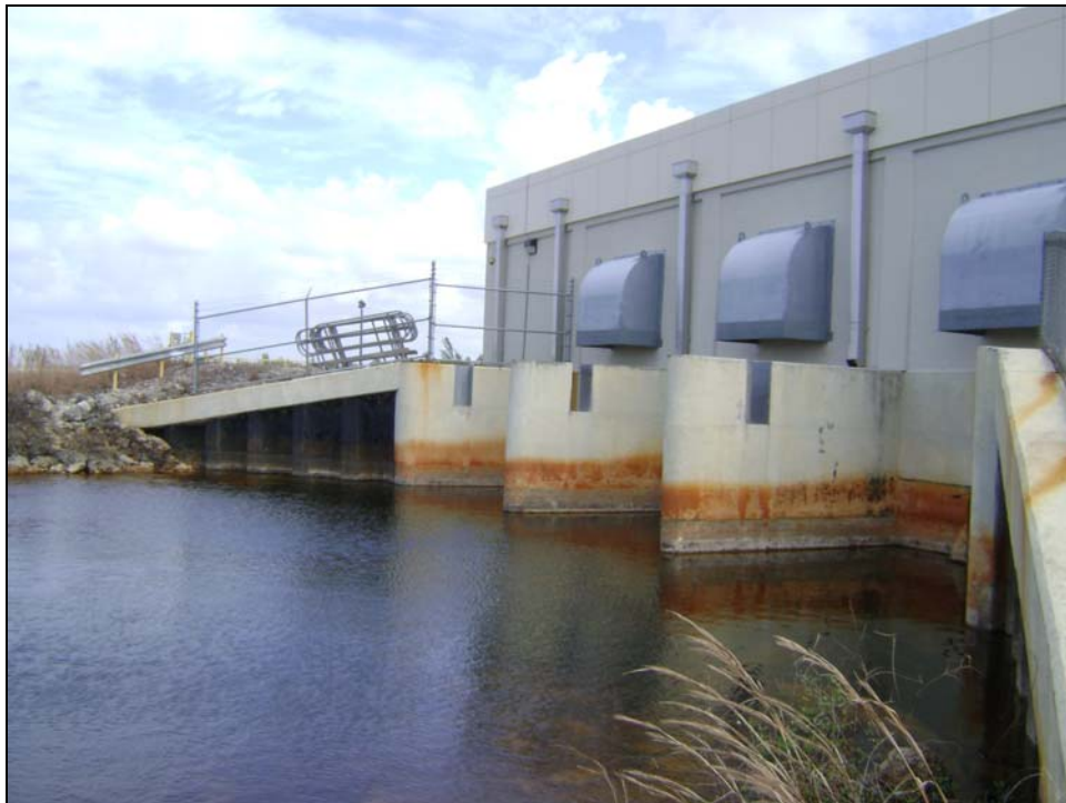
Figure 32. Northeasterly view of the G-420 Intake Pump Station showing the discharge bays. The concrete abutments and steel sheet pile walls are in good condition.
