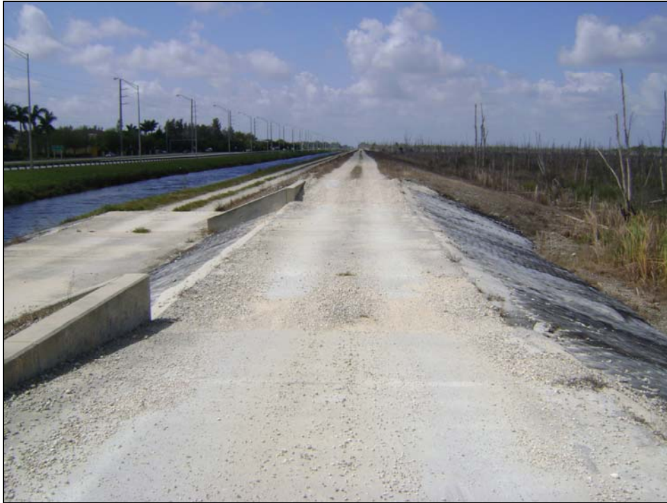
Figure 23. Westerly view of the Emergency Spillway. The concrete surface is in good condition. Some vegetation growth along the construction joints.
