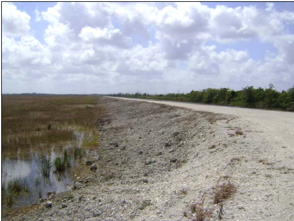
Figure 14. Southerly view of the North Cell West Perimeter Levee as seen from the northwest corner. The inside and outside slopes are 4H:1V and 1H:1V, respectively. Sparse withered vegetation noted. No ruts or erosion was observed.
