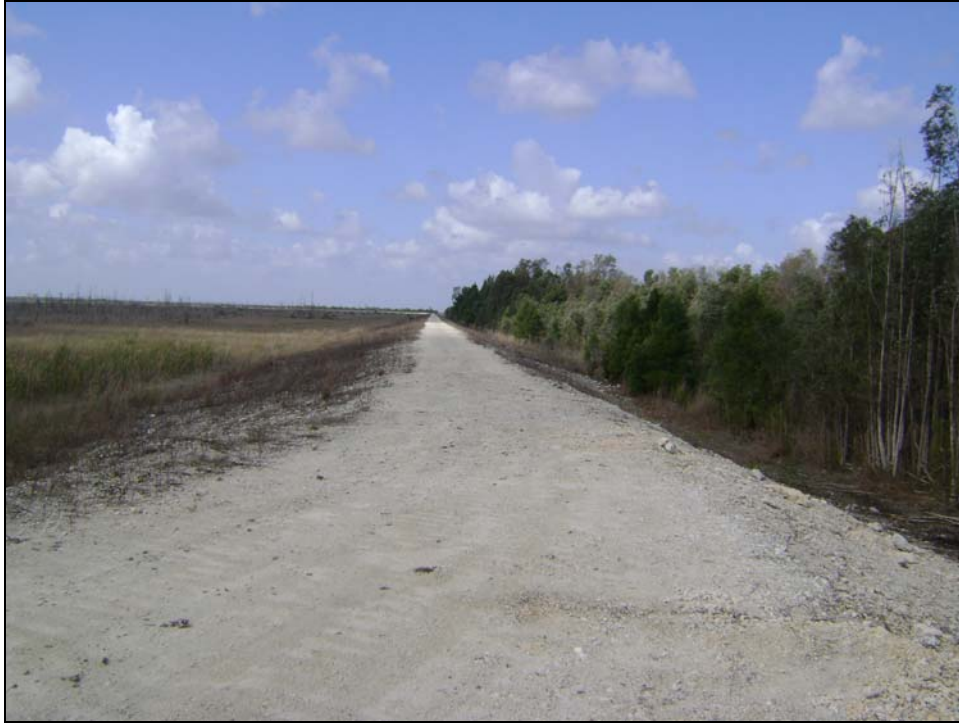
Figure 11. Westerly view of the North Cell North Perimeter Levee as seen from the northeast corner. The inside and outside slopes are 4H:1V and 2.5H:1V, respectively. Sparse vegetation noted and is withered. No ruts or erosion was observed.
