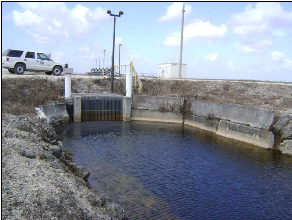
Figure 34. Westerly view of the G-420S Seepage Pump Station showing the trash rack and Jersey barrier wall.
