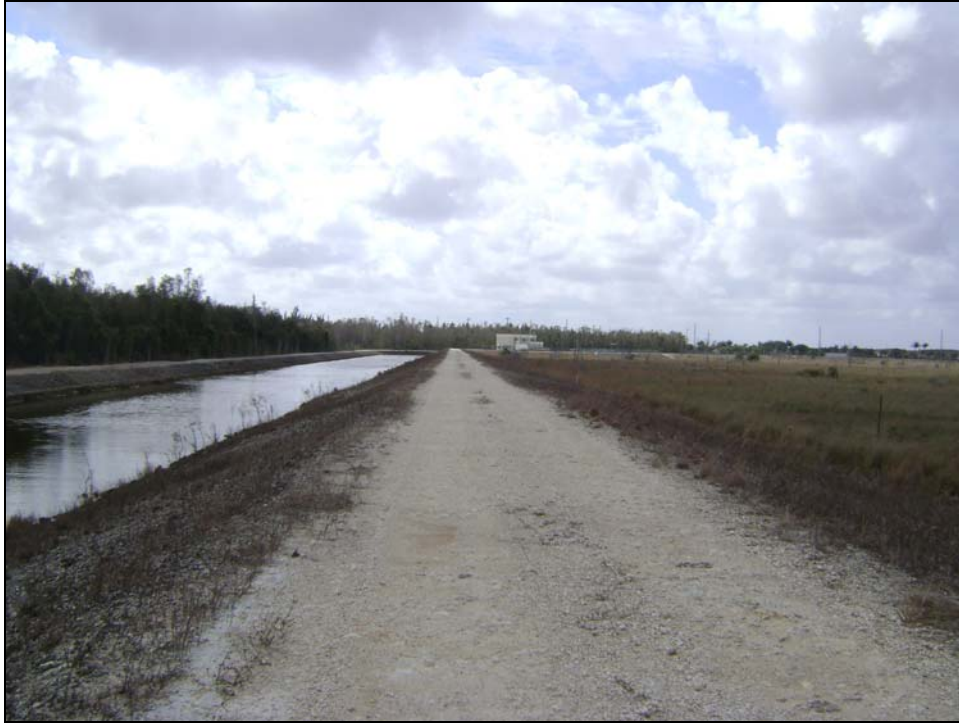
Figure 5. Southerly view of the 14-foot wide East Perimeter Levee 0.28 miles north of the G-422 Pump Station. The inside and outside slopes are 4H:1V and 2.5H:1V, respectively. Majority of the side slopes are bare of vegetation. The weeds on the slopes are withered. No ruts or erosion was observed.
