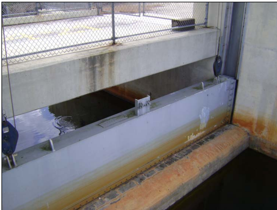
Figure 29. View of the G-421 Gated Spillway Structure vertical roller gate and weir crest.
