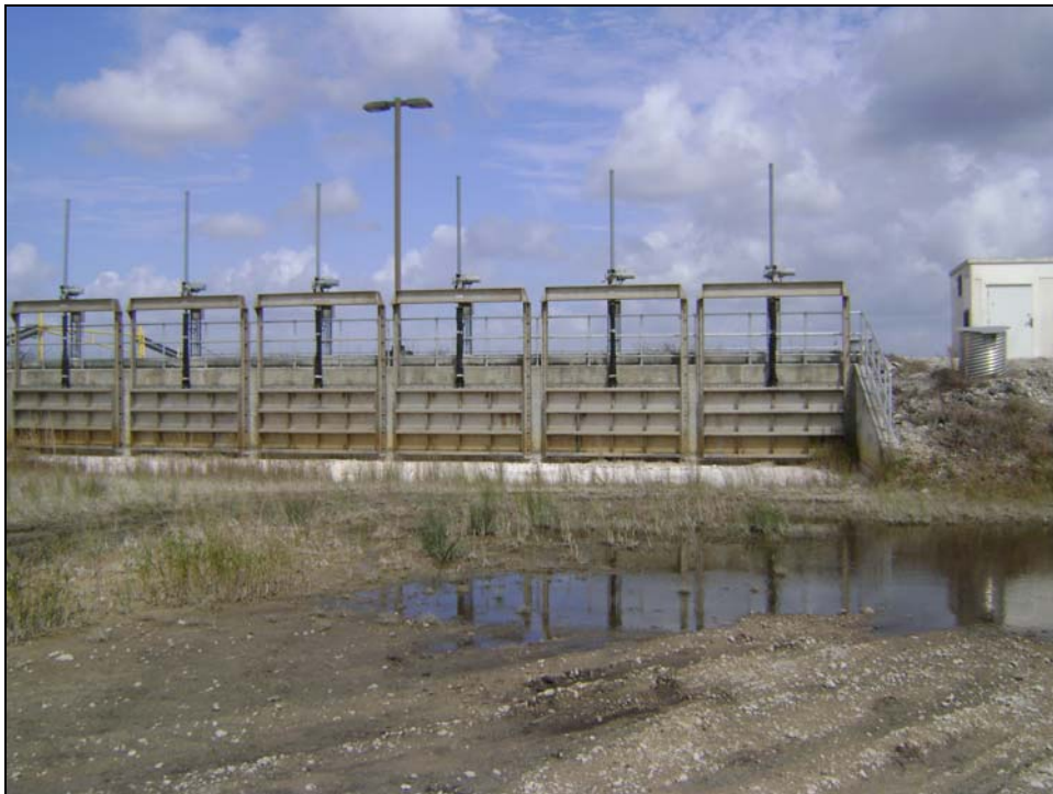
Figure 36. Northerly view of the G-423 Interbasin Transfer Structure with six 5-foot high by 10-foot wide gated culverts.
