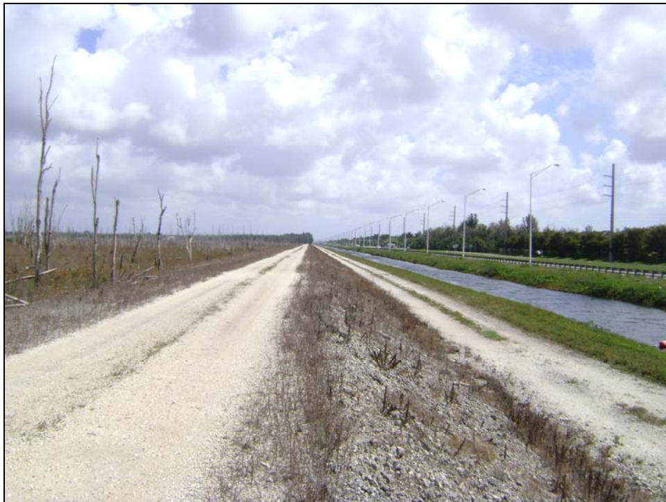
Figure 22. Easterly view of the 14-foot wide South Cell South Perimeter Levee and 25-foot wide berm approximately 200 feet east of the southwest corner. The inside and outside slopes are 4H:1V and 2H:1V, respectively. Sparse withered vegetation noted. No ruts or erosion was observed.
