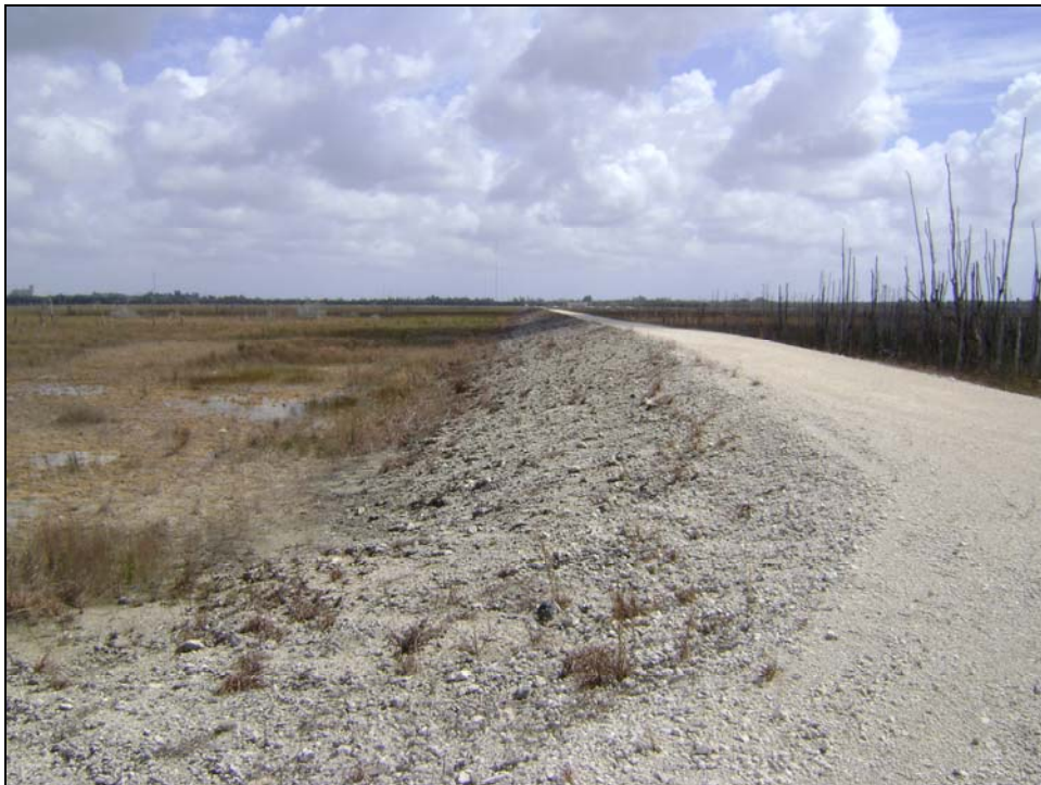
Figure 18. Easterly view of the 10-foot wide Interior Levee between the North and South Cells. The levee slope is 4H:1V. Sparse withered vegetation noted. No ruts or erosion was observed.
