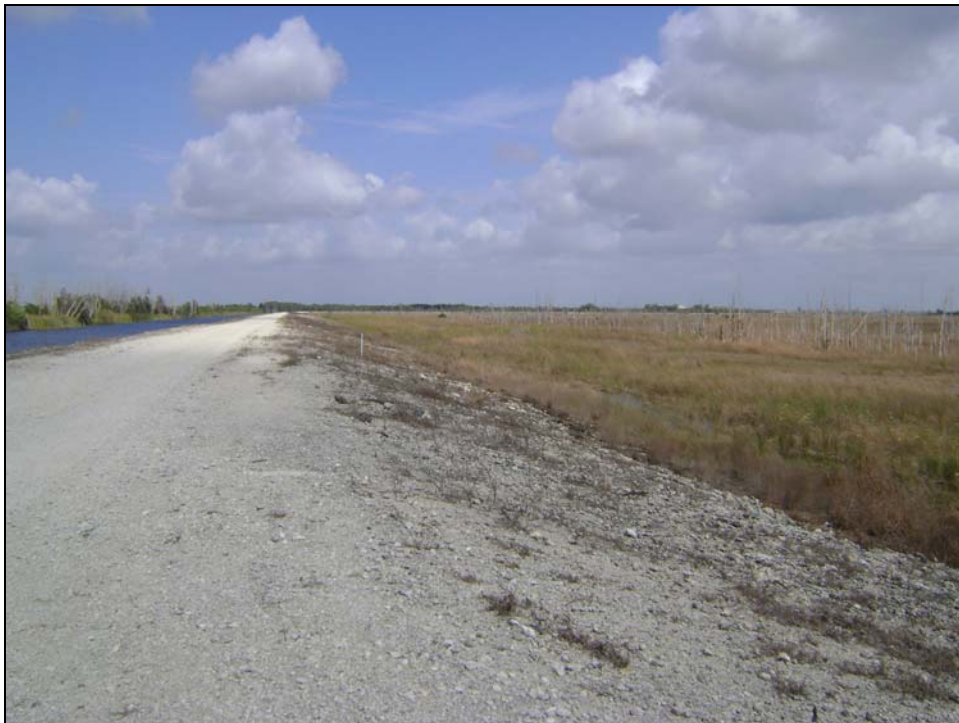
Figure 16. Northerly view of the 25-foot wide North Cell West Perimeter Levee as seen from its junction with the Interior Levee. The inside and outside slopes are 4H:1V and 1H:1V, respectively. Sparse withered vegetation noted. No ruts or erosion was observed.
