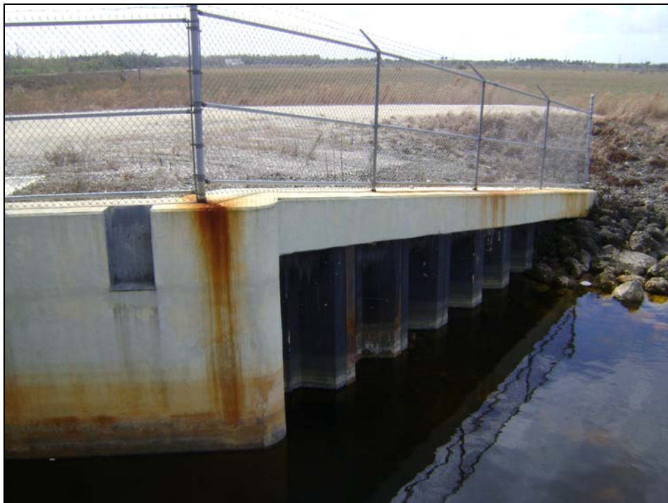
Figure 28. Southwesterly view of the G-421 Gated Spillway Structure Wingwall. Iron oxide stains from minor corrosion of fence posts. No cracks were observed on the concrete surfaces.
