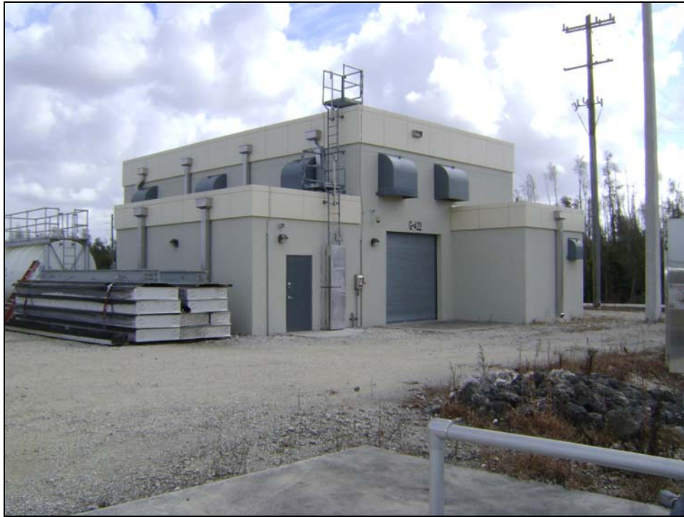
Figure 27. Northeasterly view of the G-422 Intake Pump Station Emergency Generator Building. The roof was repaired in 2011.
