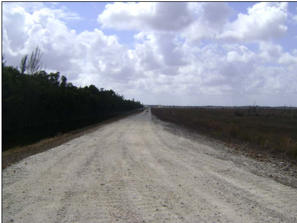
Figure 8. Southerly view of the North Cell Perimeter Levee as seen from the northeast corner of the North Cell. The inside and outside slopes are 4H:1V and 2H:1V, respectively. Vegetation on the slopes is withered. No ruts and erosion observed.
