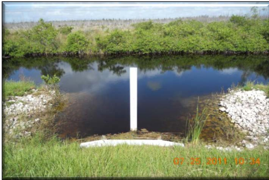
Figure 9- BBCW, L-31E Culvert S-23D upstream staff gauge.
