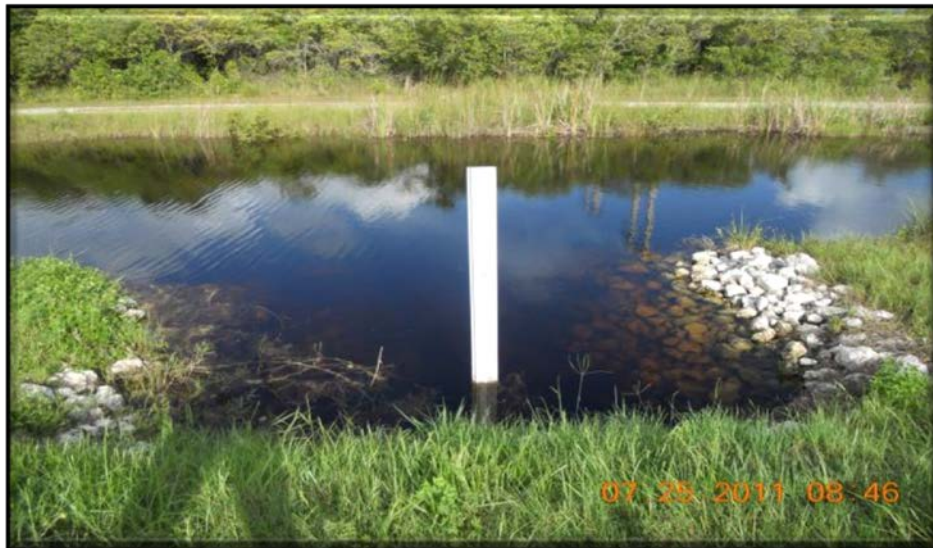
Figure 5- Biscayne Bay Coastal Wetlands, L-31E Culverts Project Staff Gauge Upstream of Culvert S-23A
