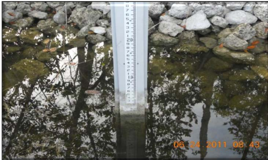
Figure 6- Biscayne Bay Coastal Wetlands, L-31E Culverts Project Staff Gauge Downstream of Culvert S-23A
