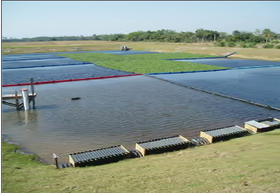
Figure 10-9. The Nubbin Slough Hybrid Wetland Treatment Technology (HWTT) facility with the mixing chamber and inflow manifold in the foreground, and the outflow riser at the upper right (photo by the SFWMD).
