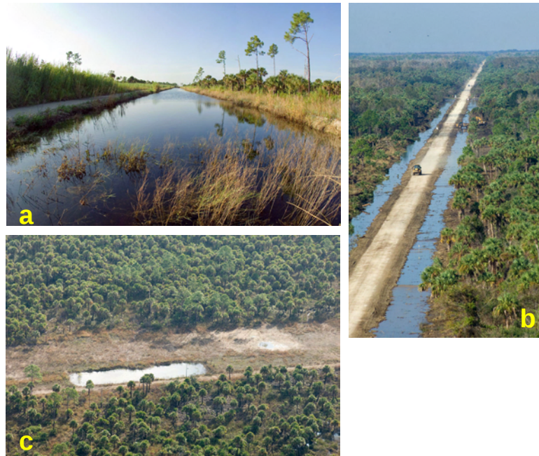
Figure 133. A Picayune Strand Restoration Project Area canal (a) before, (b) during, and (c) after filling (photos by the SFWMD).
