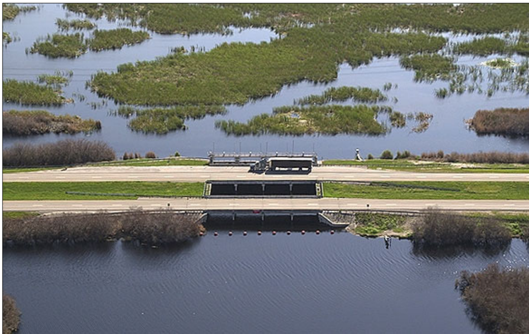
Figure 1B-8. Structure S-11B, an example of an outflow structure from WCA-2A (photo by P. Lynch, SFWMD).
