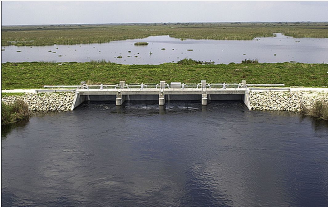
Figure 1B-7. Structure S-10A, an example of an inflow structure to WCA-2A (photo by P. Lynch, SFWMD).
