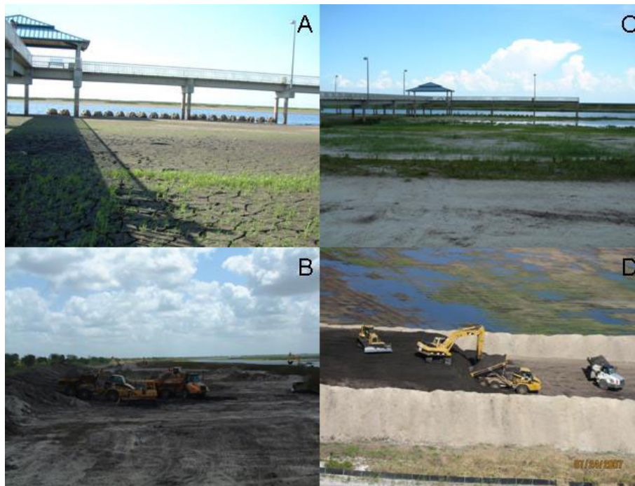
Figure 10-34. Sediment scraping project: ( Panel A ) Eagle Bay Island before sediment removal, ( Panel B ) during removal, and ( Panel C ) after removal. Panel D , disposal of material from Fisheating Bay to the C-41 canal berm.
