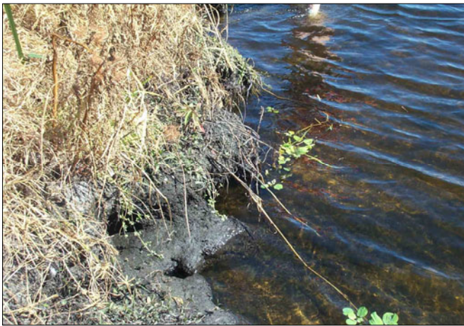
Figure 9-53. Sailfin catfish tunneling is believed to damage canals and levees and result in increased siltation (photo by USACE).
