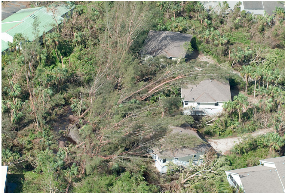
Figure 9-39. Tall Australian pine trees blocked roads, snapped powerlines, and were responsible for extensive structural damage on the coastal islands after Hurricane Charley (photo by SFWMD).
