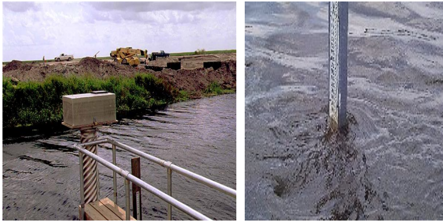
Figure 28. Stilling well and stage recorder (left) and vertical staff gauge (right).
