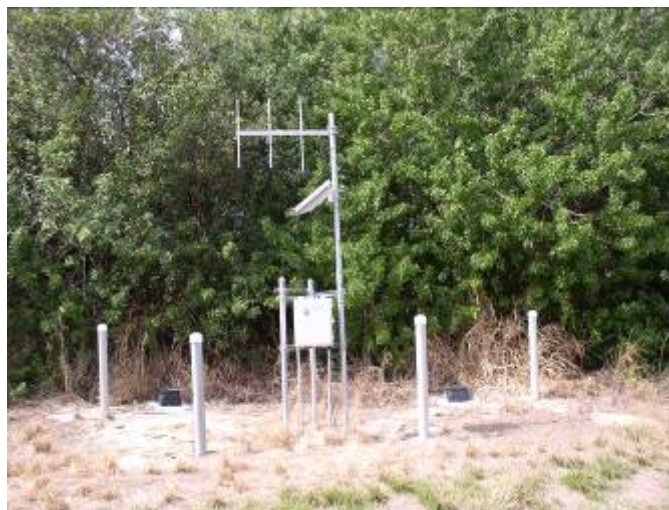
Figure 60. A non-artesian well site connected via telemetry.
